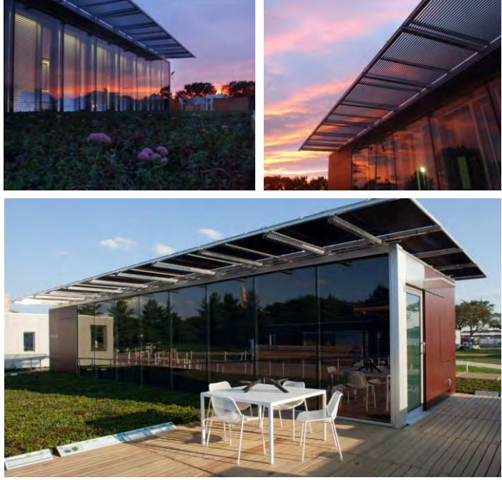
In the Living Light house the ubiquitous glass façade is re-imagined as a transparent wrapper that simultaneously resolves dissimilar interior and exterior design criteria.
