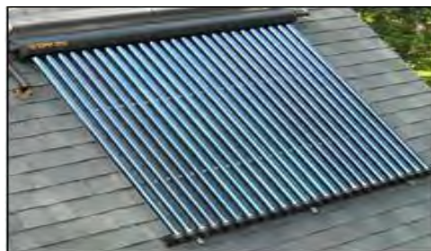
Evacuated tube solar collector
