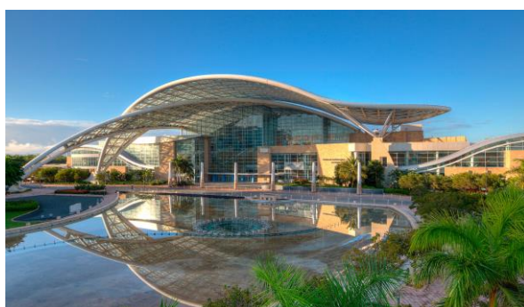
The Puerto Rico Convention Center is the largest and most technologically advanced meeting facility in the region. It's also one of the greenest!
