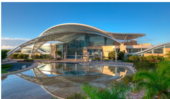
The Puerto Rico Convention Center is the largest and most technologically advanced meeting facility in the region. It's also one of the greenest!
