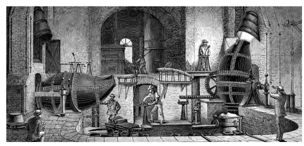
Kelly's pneumatic process, when combined with later improvements, made large-scale economical production of iron and steel in the U.S. possible during the latenineteenth century.
