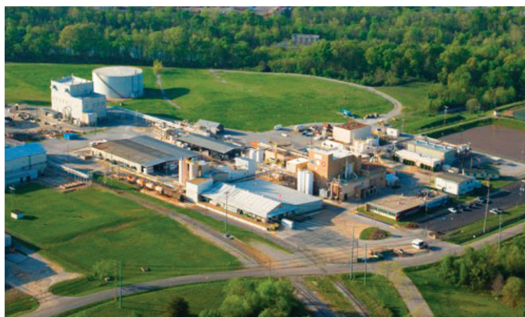
Grace produces Raney nickel at its Chattanooga, Tennessee, manufacturing plant. W. R. Grace
