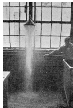
AN EMERGENCY SHOWER SHOULD ALWAYS BE HANDY IN ANY LABORATORY WHERE SMALL-SCALE OPERATIONS ARE TRIED OUT
