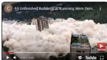
15 Unfinished Buildings in Kunming Were Demolished by Blasting, 1...
