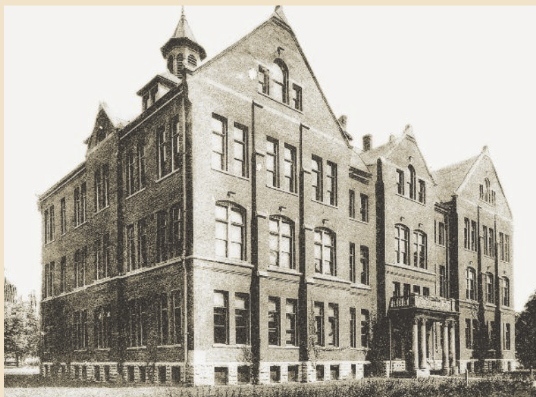
In 1901, DePauw University received a gift of $25,000 from D. W. Minshall to construct a new science laboratory. Phillip S. Baker, the first DePauw Professor of Chemistry, did much of the planning for this building. Minshall Laboratory was completed in the spring of 1902. It was demolished in 1973.
