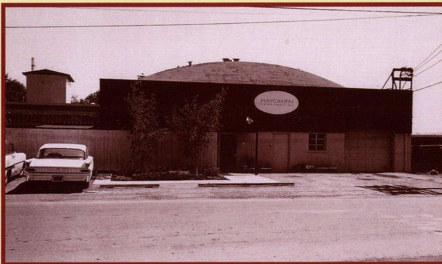
The first Raychem site at 2821 Fair Oaks Avenue in Redwood City, California. The small rectangular building at left houses the original electron beam.
