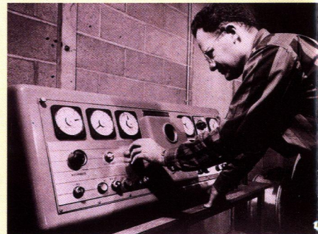
Raychem co-founder Richard W. Muchmore at controls of GE resonant-beam generator.
