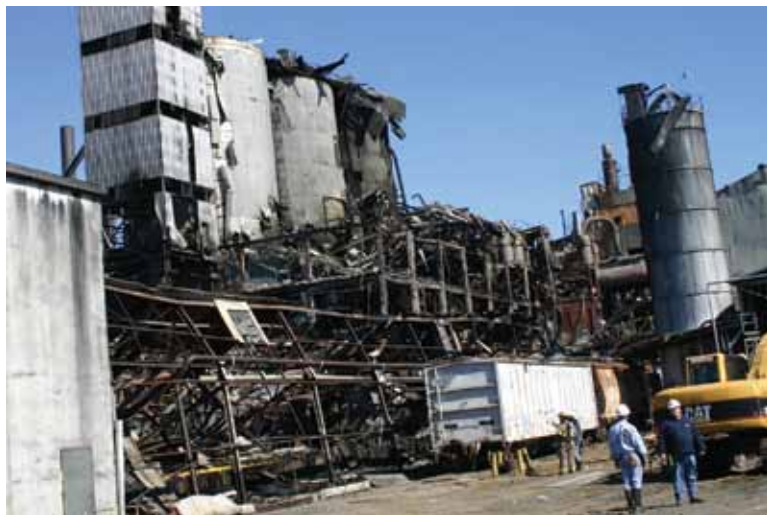
Investigators and firemen at the site of the explosion and fire at the Imperial Sugar Refinery in Port Wentworth, Ga.
