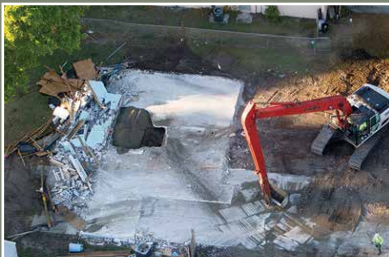
This aerial photo shows workers picking up remnants from a home in Seffner, Fla. A huge sinkhole opened under the bedroom in this home and swallowed the owner, Jeff Bush.
