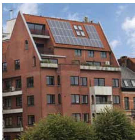
Figure 1. Solar cells are arranged in the form of a module, which are then combined to form an array. A solar panel, such as the one shown on the roof of this house, consists of a series of arrays that are aligned next to each other.
