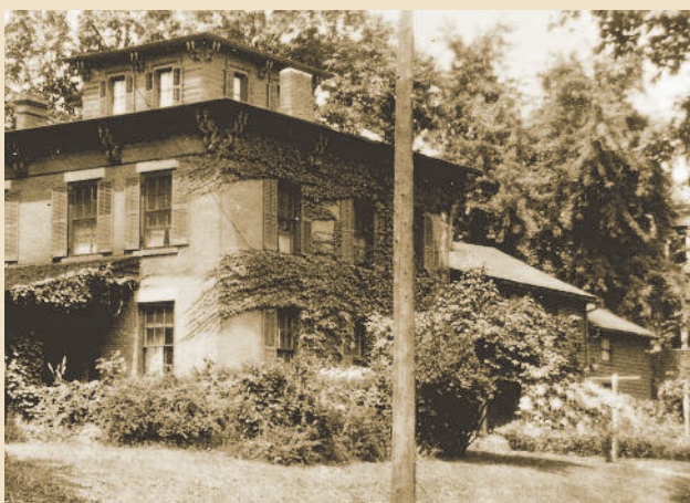
Hall family home with attached woodshed.
